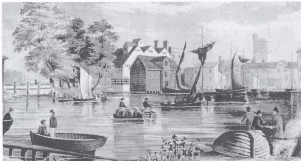
Figure 6 depicting the activity and buildings at the Town Quay in 1832 with St Margaret's in the background (source: Tames Barking Past page 59)
