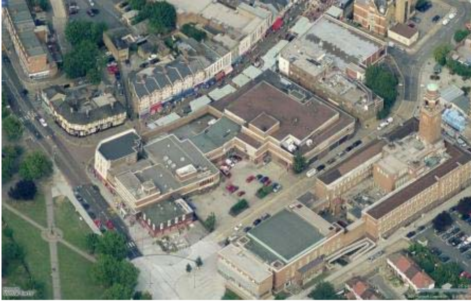
Figure 38 aerial photo of the civic quarter comprising of the Town Hall and Broadway Theatre and shows that including no.s 10-32 East Street in the centre of the photo as a negative contributor is important otherwise they will be an island isolated in the middle of the conservation area (source: Bird Heritage Scoping study Design for London)
