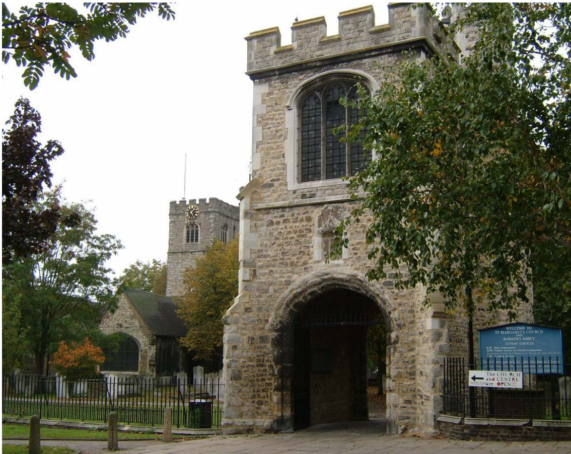
Figure 1 of the Curfew Tower and St Margaret's Church in the Abbey and Barking Town Centre Conservation Area (source: the writer)
